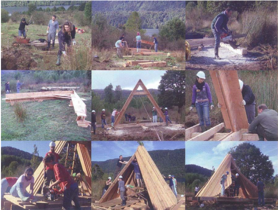
Figure 79: Construction process of shelter & viewing platform. (Source: Hensel M. et al 2010)
