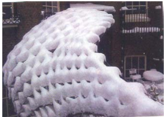
Figure 68: AA Canopy exposed to severe snow loads. (Source: Hensel M. et al 2010)
