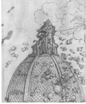
The lantern being struck by lightning in 1601, and the scaffolding erected to repair it.
