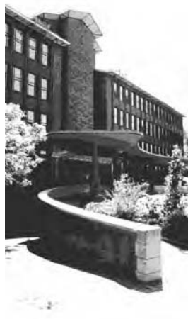
Figure 6.1 Former KLM head office, Plesmanweg, The Hague (Binnekamp, 1995, p. 1)
